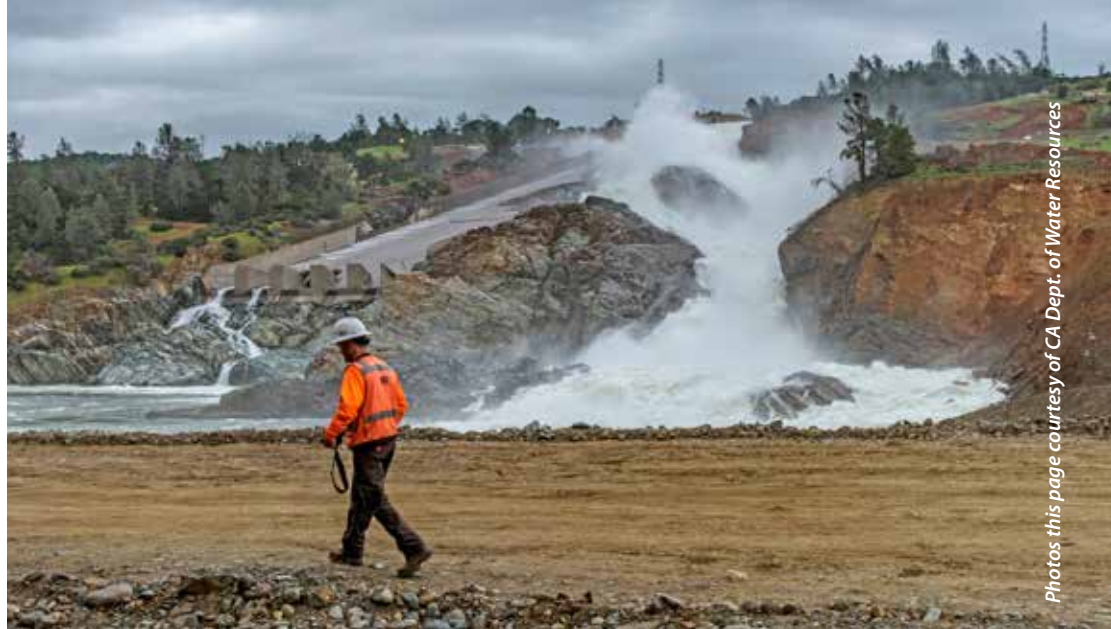
Water rushes into the diversion pool from the ravine carved out from the damaged Lake Oroville spillway. Photo taken April 26, 2017. Learn about our connection to Lake Oroville at www.dsrds.com/oroville .
