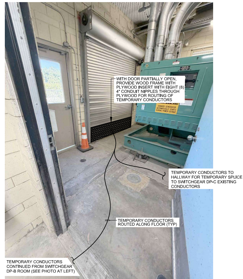
DOORWAY BETWEEN SWITCHGEAR DP-B ROOM AND GENERATOR ROOM
