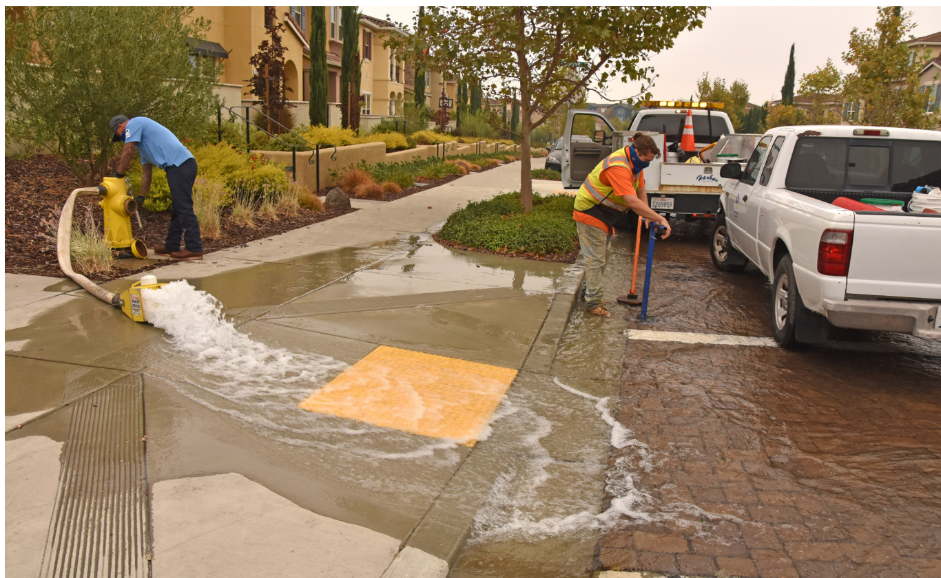
Scheduled hydrant flushing maintains water quality.
