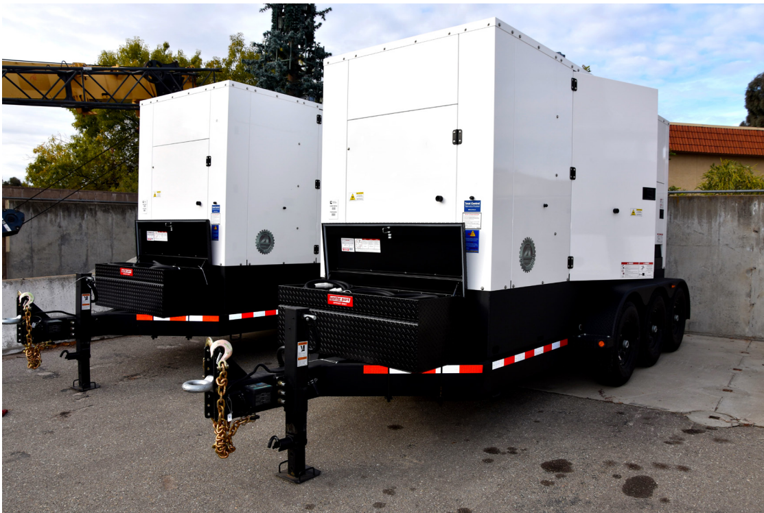
Two 275kW portable standby generators for the Potable Water Pump Station Emergency Response CIP.
