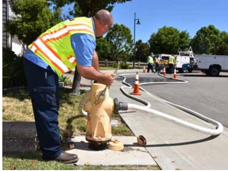
*Water/Wastewater Systems Lead Operator Danny Leonardo opens the hydrant used to flush a drinking water main.*
