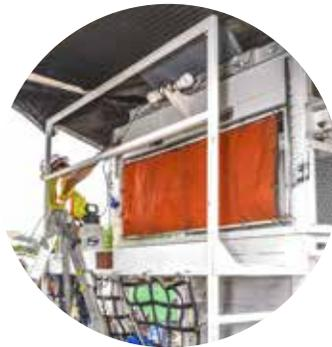
*The liner is temperature sensitive and shouldn't be exposed to high heat. A shade canopy shields it from premature fusing before installation.*
