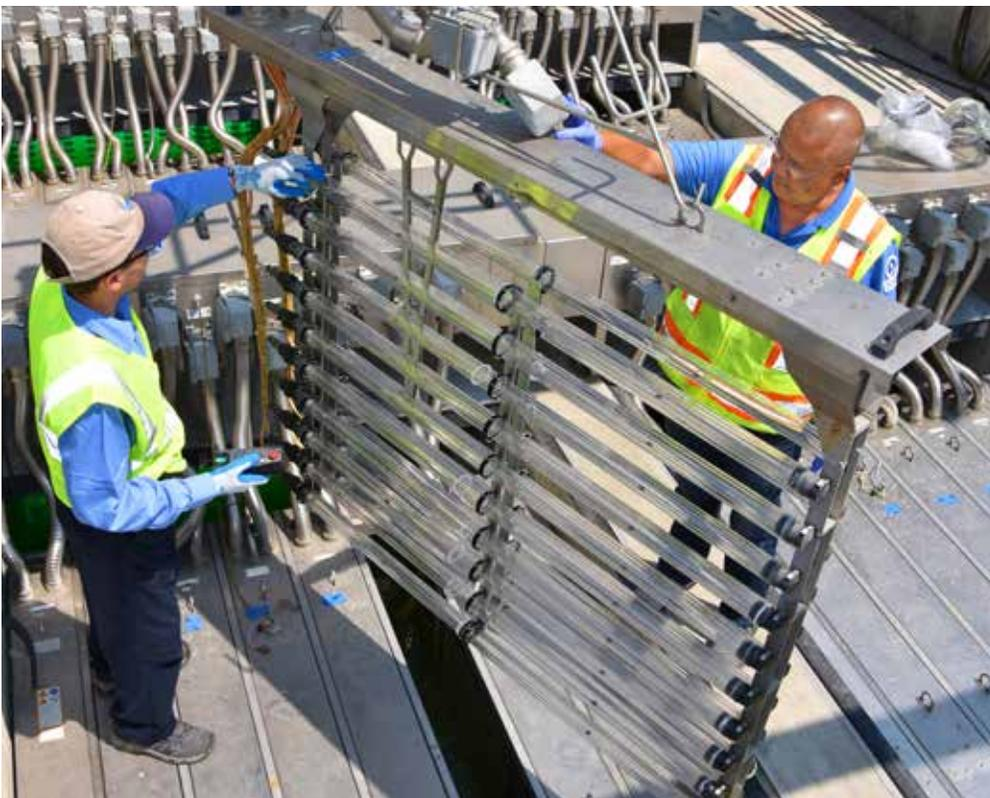
(L to R) Stephan Kozanda, Senior Wastewater Treatment Plant Operator III, and Virgil Sevilla, Process Lead Wastewater Treatment Plant Operator V, inspect ultraviolet lamps of one of the new UV modules installed during the plant expansion. In total, there are ten UV banks with seven UV modules each, totaling 1,400 UV lamps that operators inspect monthly.
