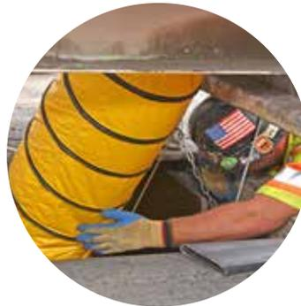
*A worker positions the forced air heating duct, which assists in curing the pipe liner.*
